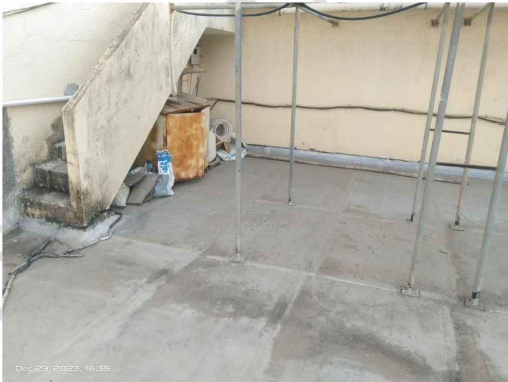
Plate 5: Space below the rooftop solar panel
